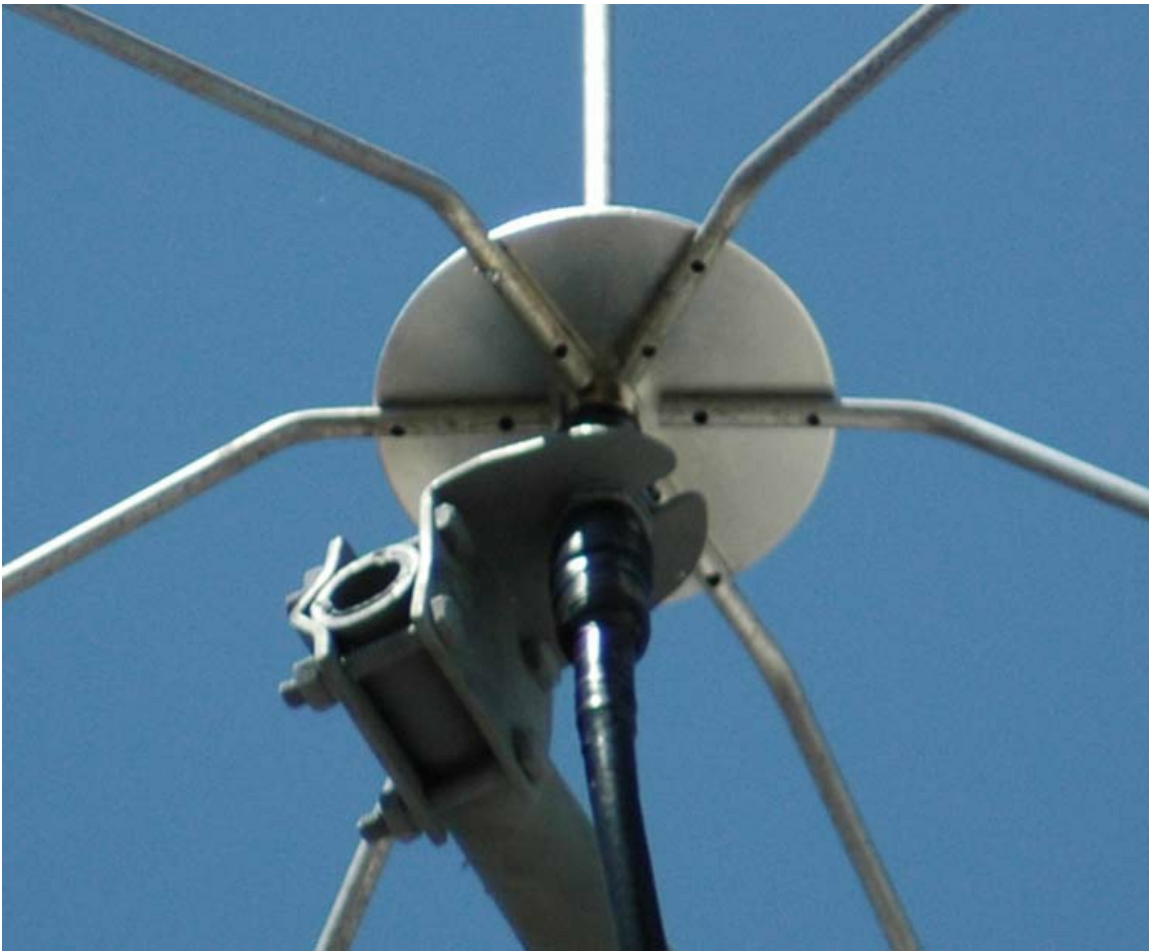
Photo 6 146MHz 1/4\lambda ground plane installed and showing mounting details.
