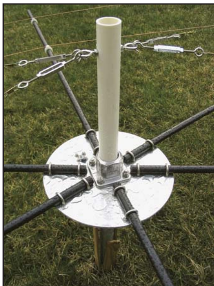
Figure 2 —A top view of the antenna center hub during construction, together with the guy anchor post.
