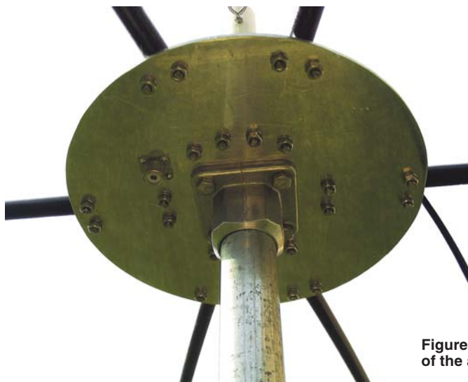
Figure 2 —A top view of the antenna center hub during construction, together with the guy anchor post.
