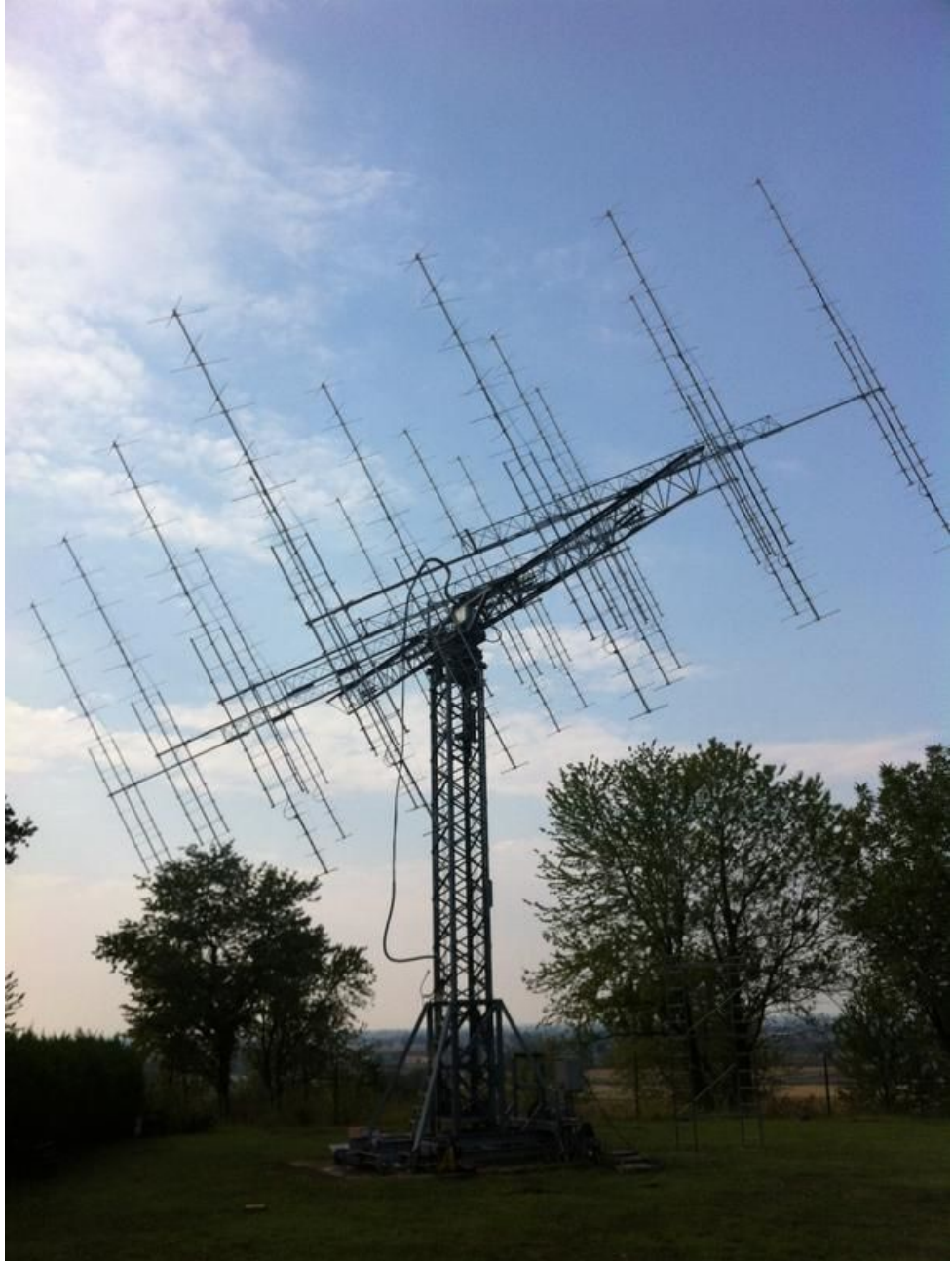
Fig. These are the EME antennas of Franco Giorgi, I2FAK. It is an Array of 16 Log-Loop Yagi of 19 elements.
