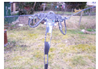
At the top of the feeder, after weather-proofing - not pretty but waterproof!!
